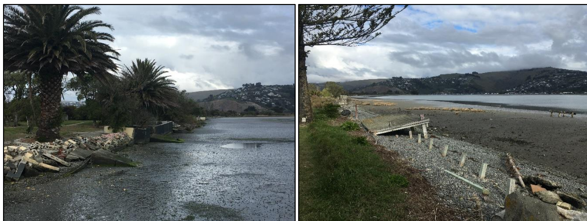
Figure 3.9: Example of informal, non-consented structures along the Avon-Heathcote Estuary.
