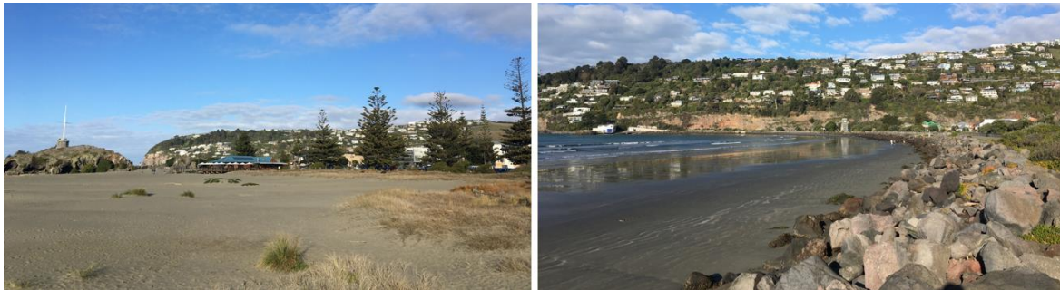
Figure 4.16: Site photos (taken August 2020) for the Sumner shoreline. (Left) unprotected dunes along Clifton Beach (Cell 28), (right) rock revetment along Sumner Bay with Sumner Headland in the background (Cell 29).
